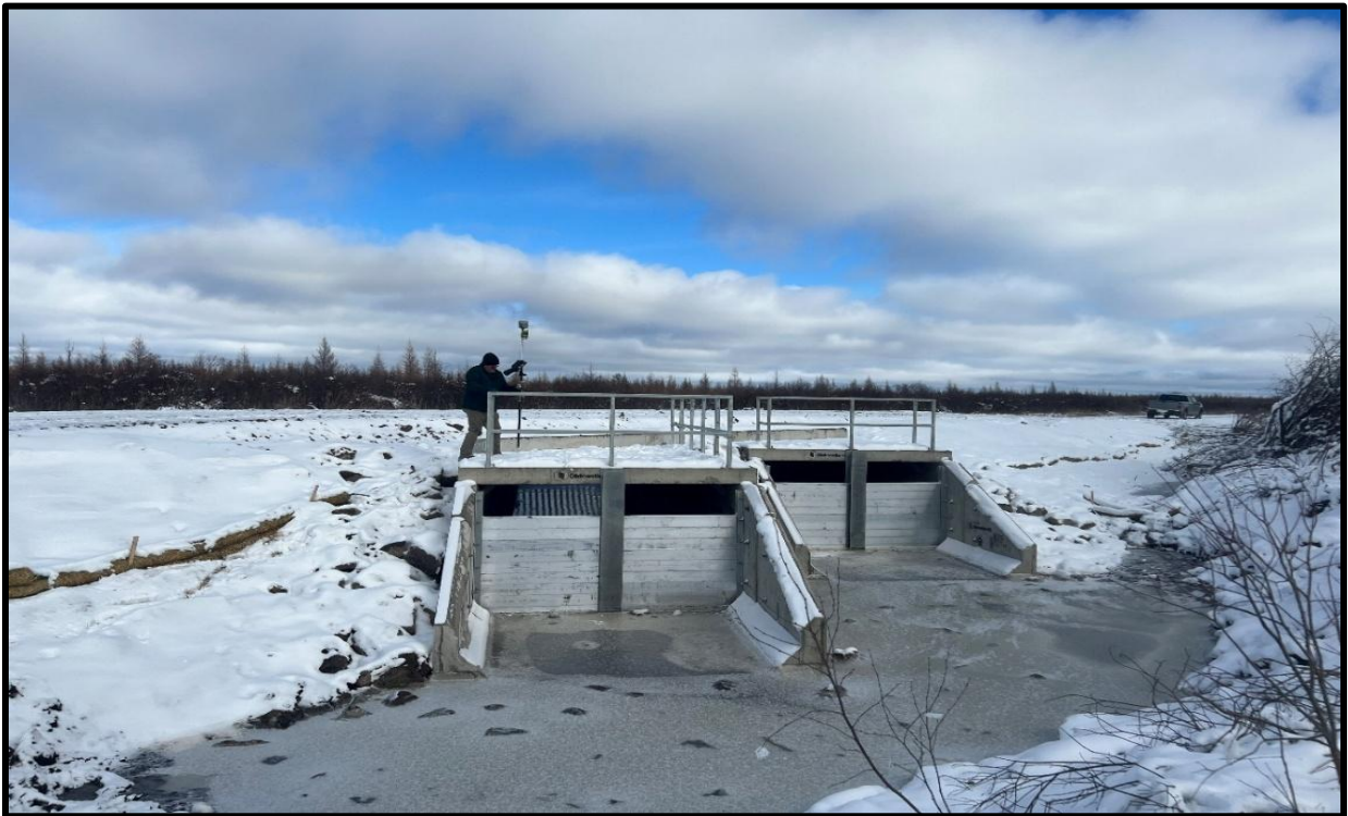
Lost River State Forest – Centerline Box culverts
