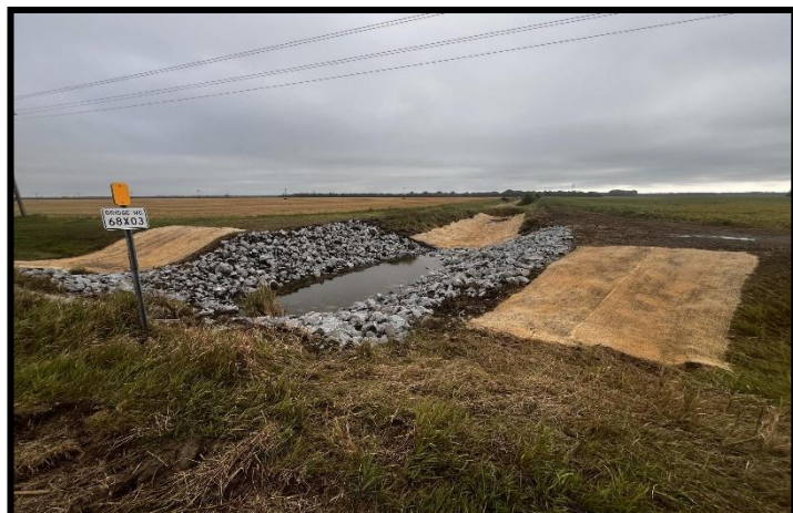
CD8 Installed riprap armoring at the centerline box culvert under HWY 89.
